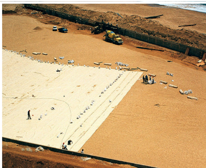
FIGURE 4: CRYSTAL LAGOONS LINER INSTALLATION
